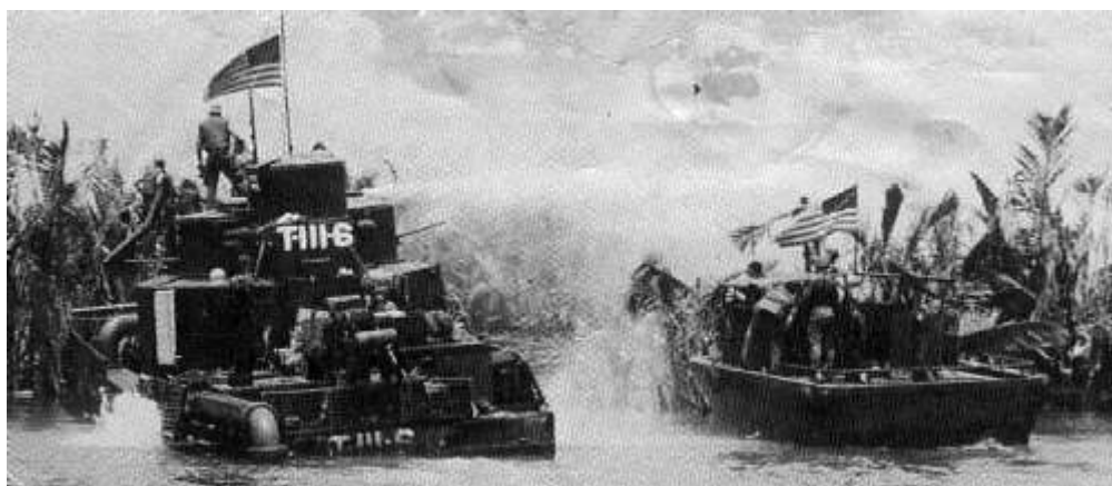
A MRF water monitor. This craft was used to destroy tunnel entrances at the river/canal bank.
